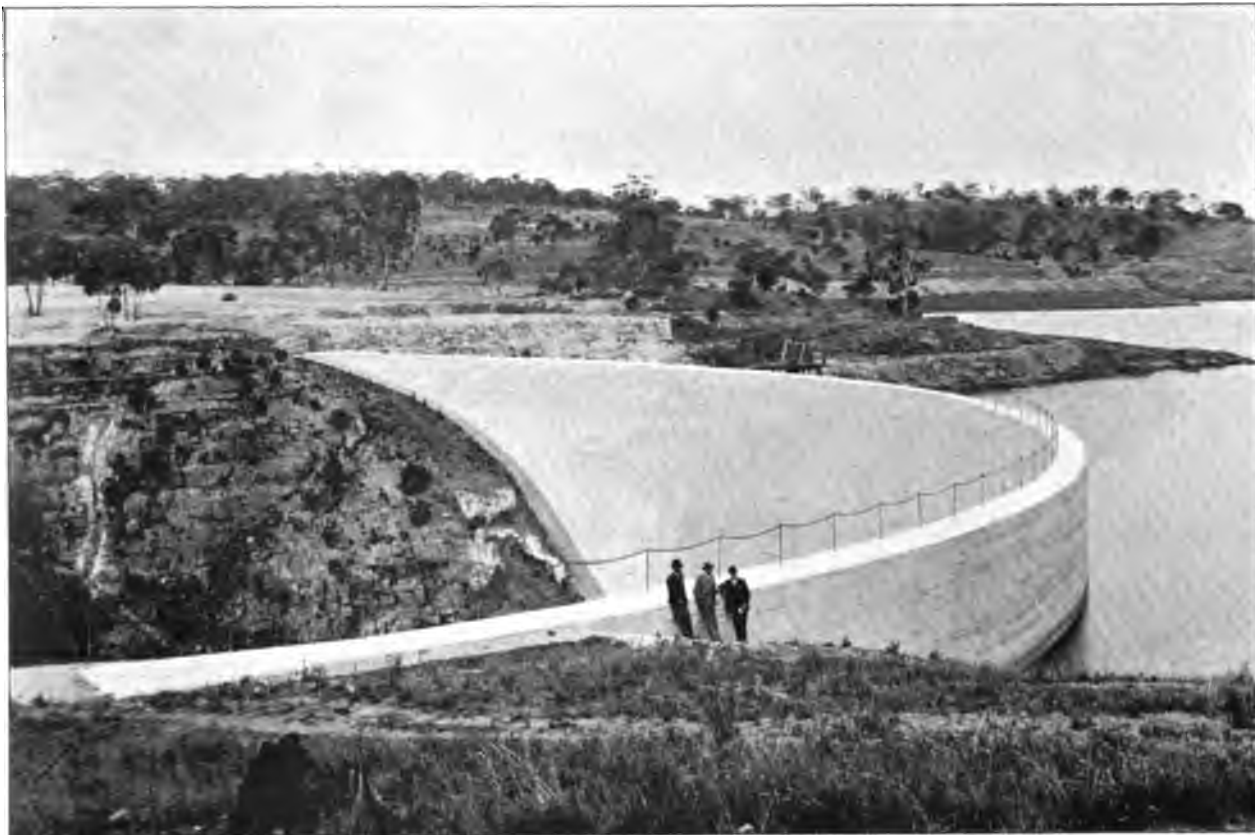
CURVED WALL. BAROSSA DAM.
